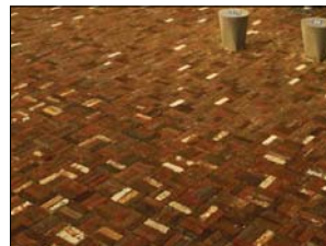
4. Recycled brick paving
